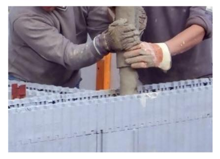
Please note, the rubber tube of the concrete pump should be reduced to 70mm diameter, 100 mm is possible, 125 mm makes it difficult.
